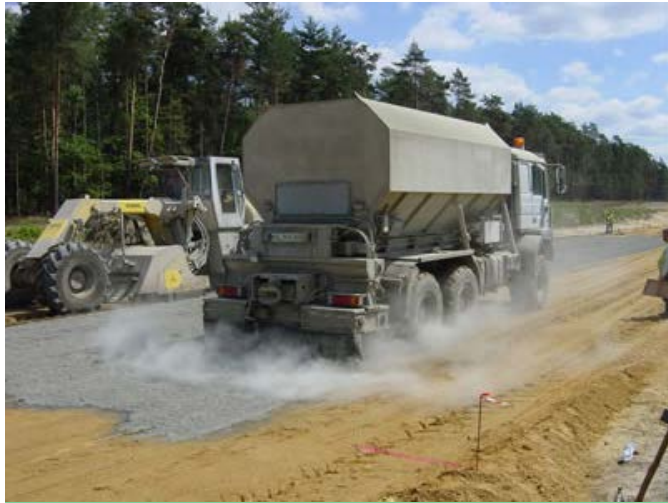
Spreader and cold mixing machine
