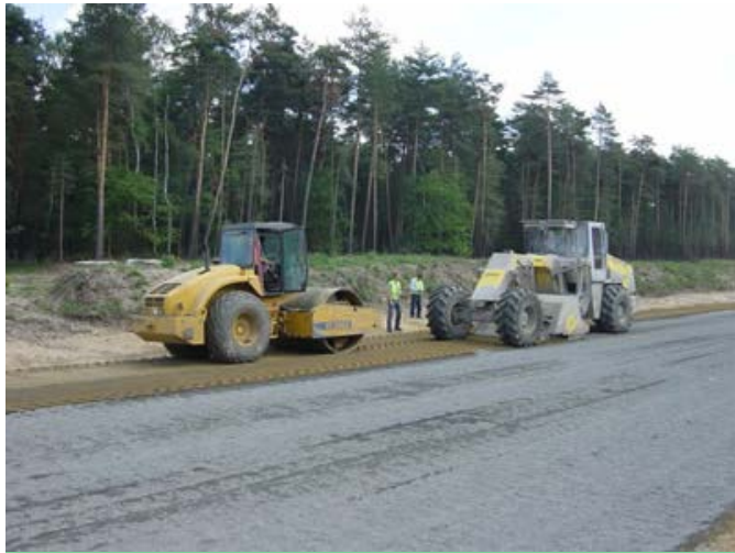
Road roller train and cold mixing machine
