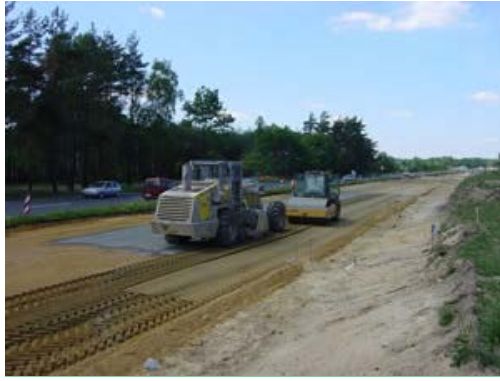
Cold mixing machine with road roller train
